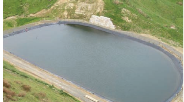
RAW WATER STORAGE DAM - MOKAU
