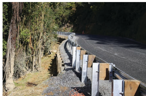
SLIP REPAIR - MANGARINO ROAD
