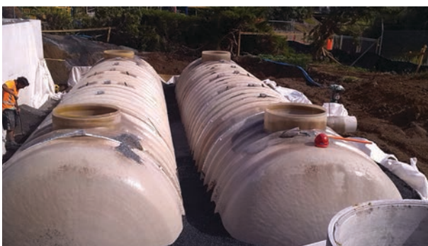
NEW WASTE WATER TREATMENT PLANT TANKS
