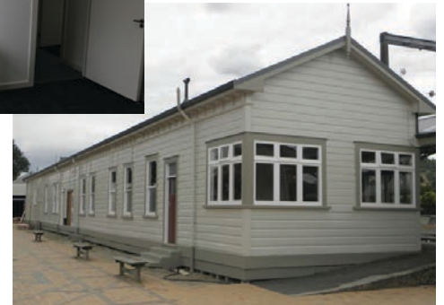
EXTERNAL WORK BUILDING 2
